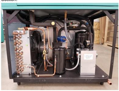
Figure 2-8 Air Cooled Condensing Unit
