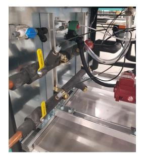
Figure 2-6 Water Cooled System Connections
