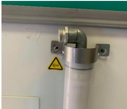
Figure 6-3 Remove the Brackets
