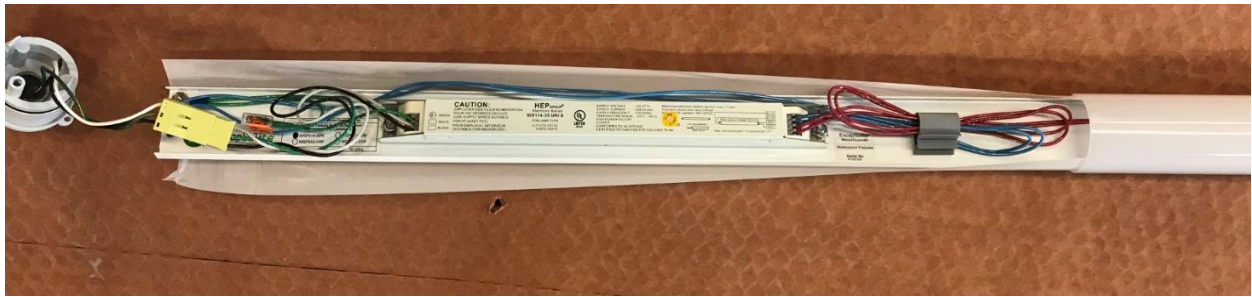
Figure 6-6 Slide the Lamp Fixture Into the Tube
