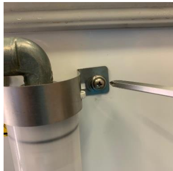
Figure 6-13 Install the Brackets
