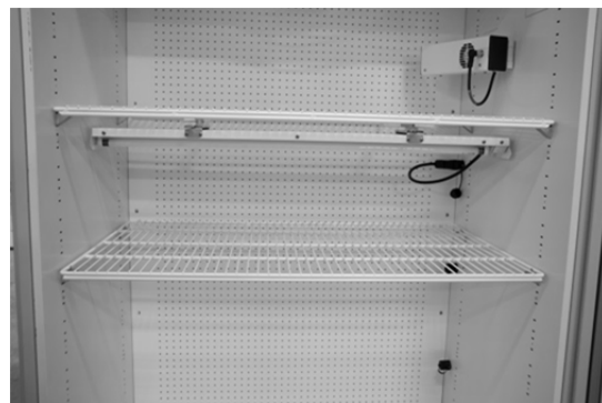
Figure 2-29 IN Single Lamp Fixture per Shelf Installed
