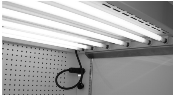
Figure 2-35 AR Lamp Canopy Installed
