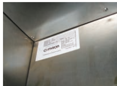
Figure 2.25: Shows in detail the back plenum installed above the fan housing.
