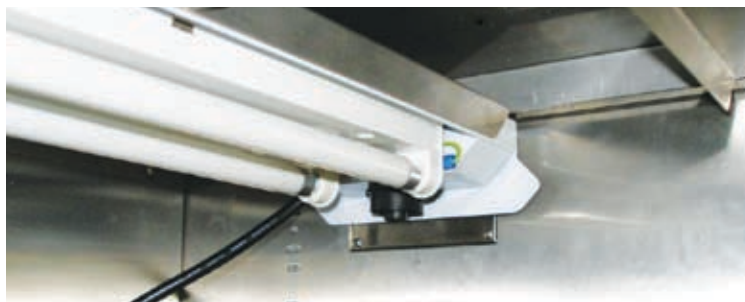
Figure 2.16: Back lamp fixture installed. (Notice the thumb screw at the front.)
