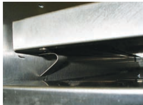
Figure 2.5: Detail of bottom self support.
