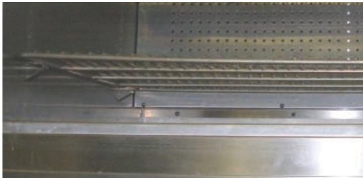
Figure 2.44: Bottom wire shelf. Notice the position with respect to the back wall plenum.
