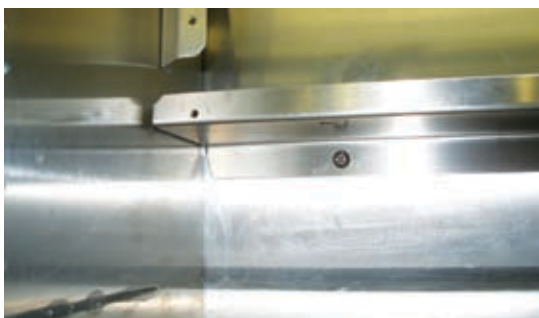
Figure 2.40: A1000 view after installing the back plenum bottom panel.
