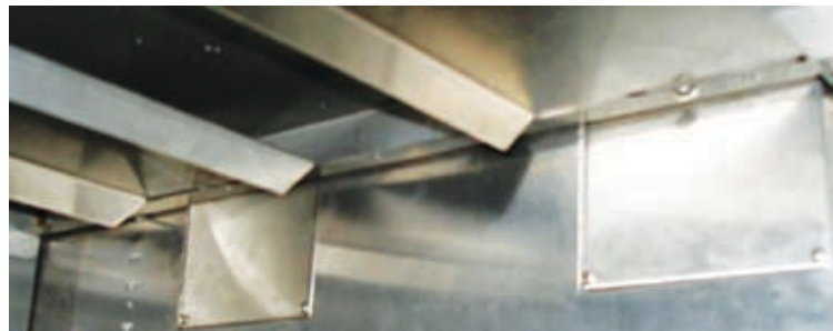
Figure 2.15: Lamp fixture supports installed.
