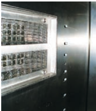
Figure 2.22: Canopy air inlet filter is showed.
