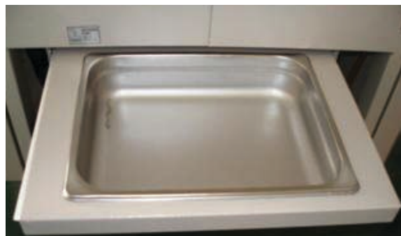
Figure 4.5: Complete drain pan installation.
