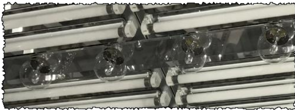
Figure 5-7: Fluorescent and Incandescent Lamp Combination
