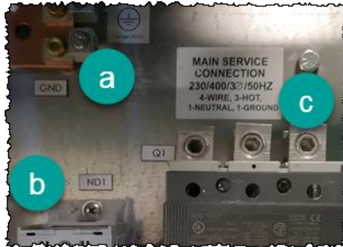
Figure 3-2: Wiring Connection Order
