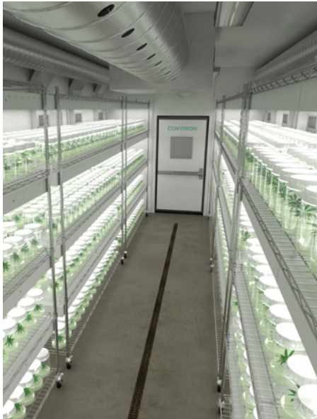
Cannabis One™ Tissue Culture Room Controlled downward airflow returning uniformly across each shelf
