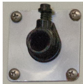
Figure 3.7: CAC Strain Relief Collar
