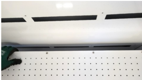
7. Insert Air Shelf metal into TC Plenum slots.
