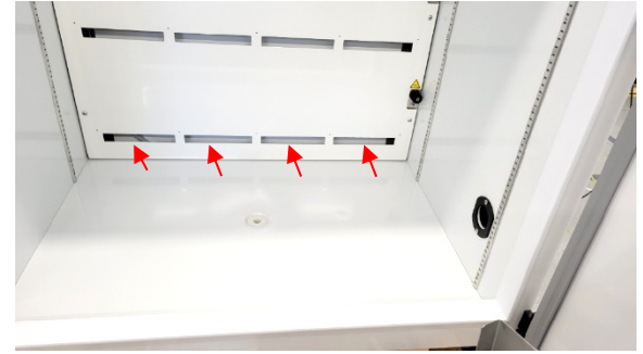
6. Line up metal from Air Shelf with slots in TC Plenum.
