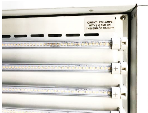
Figure 6-1 LED Tube Orientation
